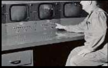
switch control center
