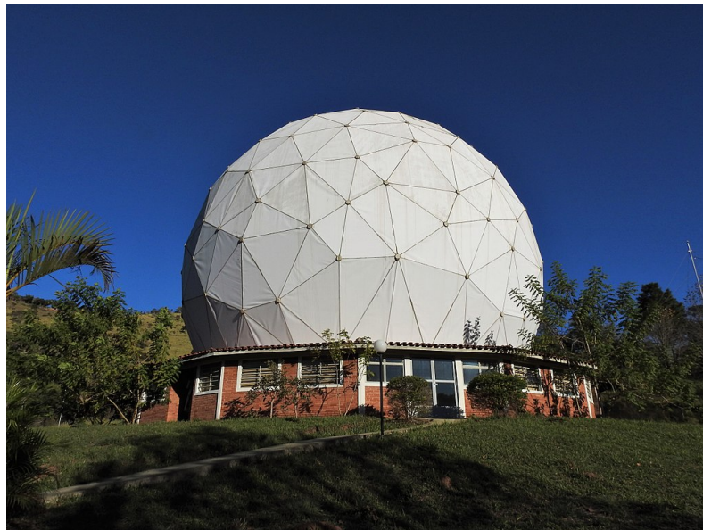
Figure 2.2: Discretization of the surface of a radio telescope in Itapetinga, Brazil [11].
